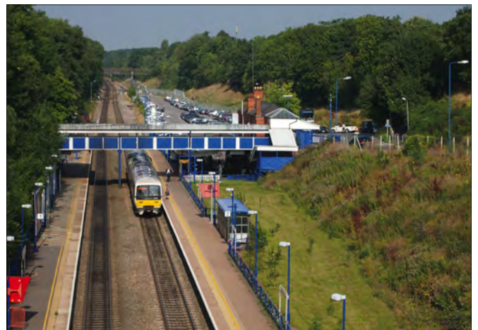
Fig 2.2: Gerrards Cross Station.
