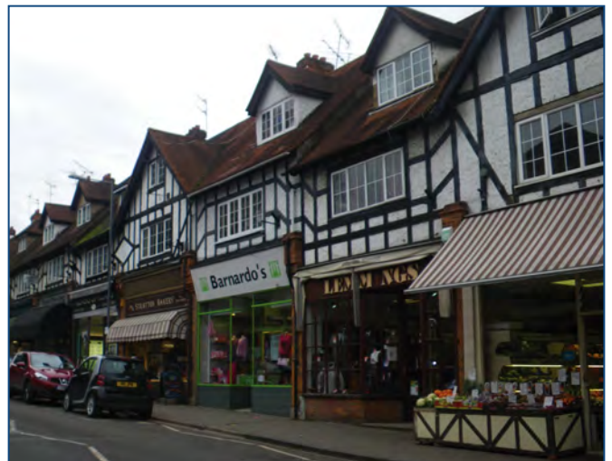
Fig 5.2: Group of buildings on Market Place.
