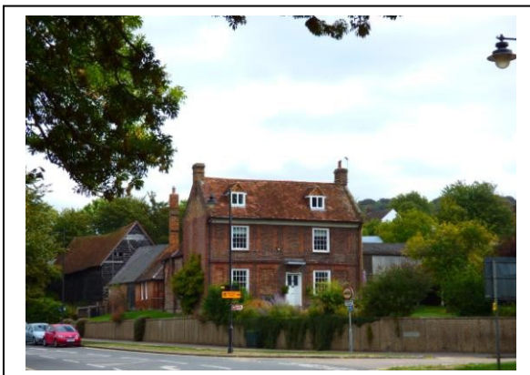
Bank Farm, Tring Rd
