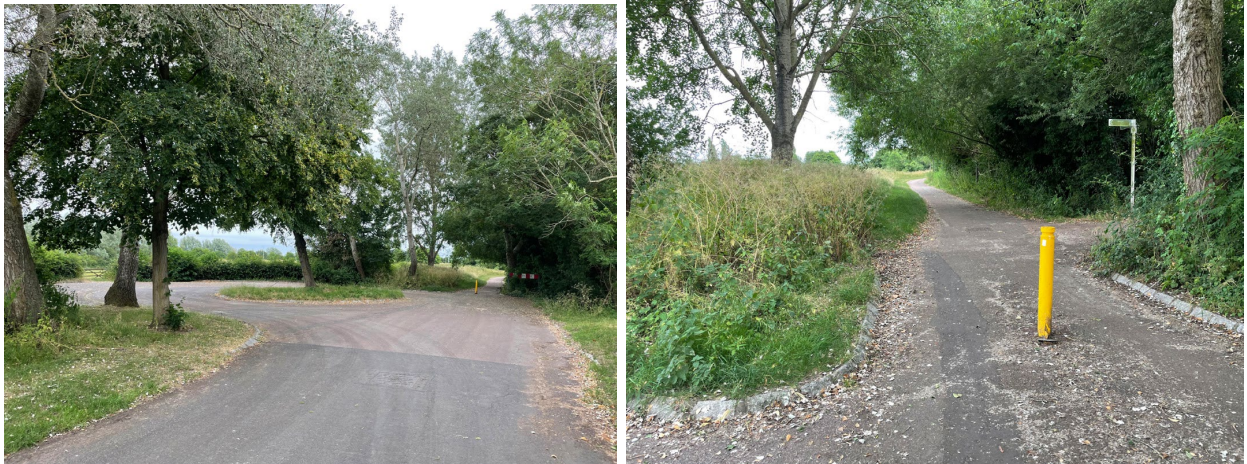
Figure 13: Photos of Stopped up route retaining landscape/vehicular access controls ('Before and after' image)
