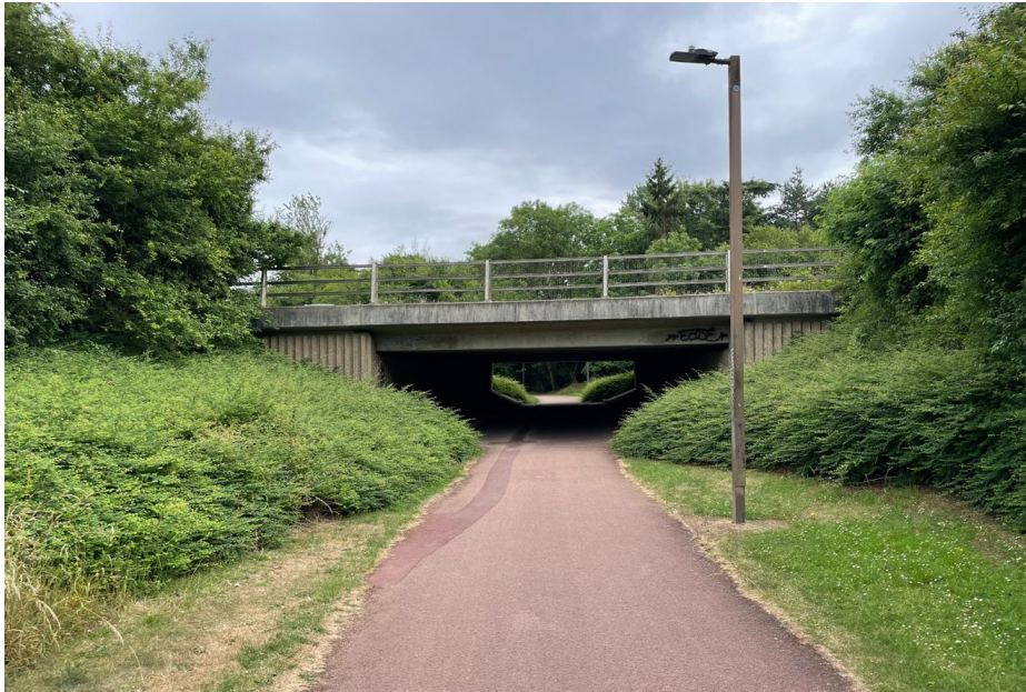
Figure 46: Example underpass in MK (lit, direct and through visibility evident)
