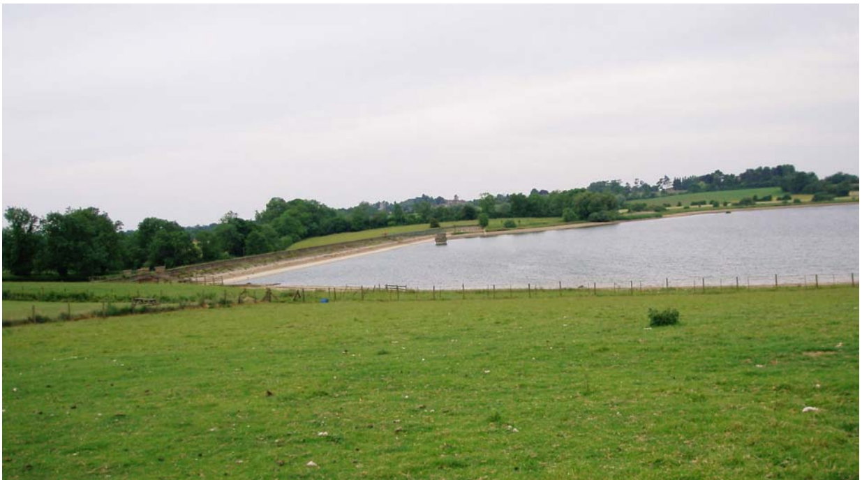
Looking south westwards across the dam of the reservoir.
