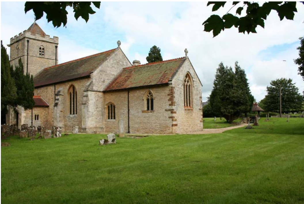
Leckhampstead Church is built of limestone which is a distinctive feature of many buildings in the area.
