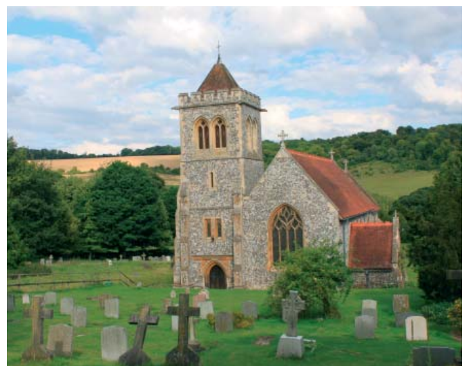
Traditional materials include brick, flint and red slate, such as at St Michael and All Angels Church at Hughenden Manor.
