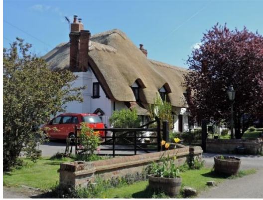
Queensmead Buckland Village
