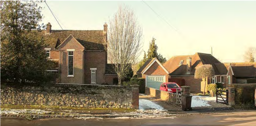
Photo 8: Lower Church Street: mixed mid-20 th century houses on larger plots with off street parking.
