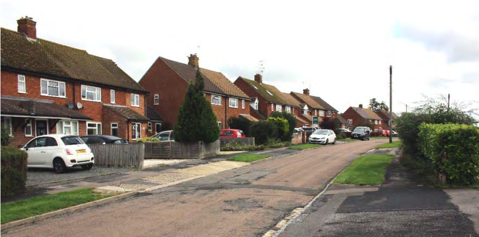
Photo 4: Bernard Close. Well-spaced houses set back from road, generous verges and off-street parking. Note loss of some verge with front gardens given over to parking – a balancing act. Overhead telephone lines are visually intrusive.
