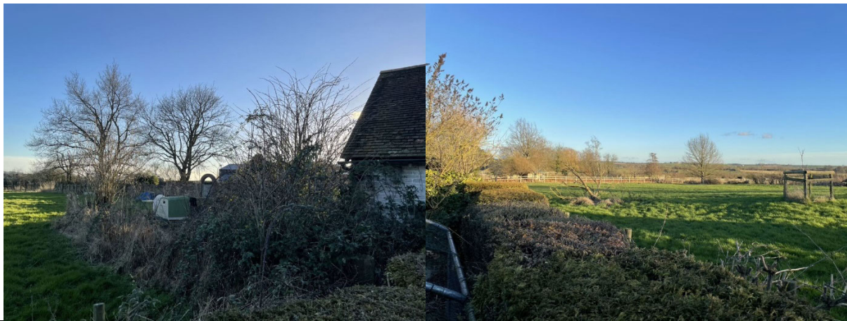
Fig.5 Outbuilding, fence and wall along the western shared boundary with Grange Farm. (Date of photo 27 Jan 2022)
