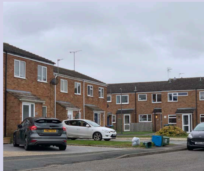
Medium density terrace housing within Stoke Grange
