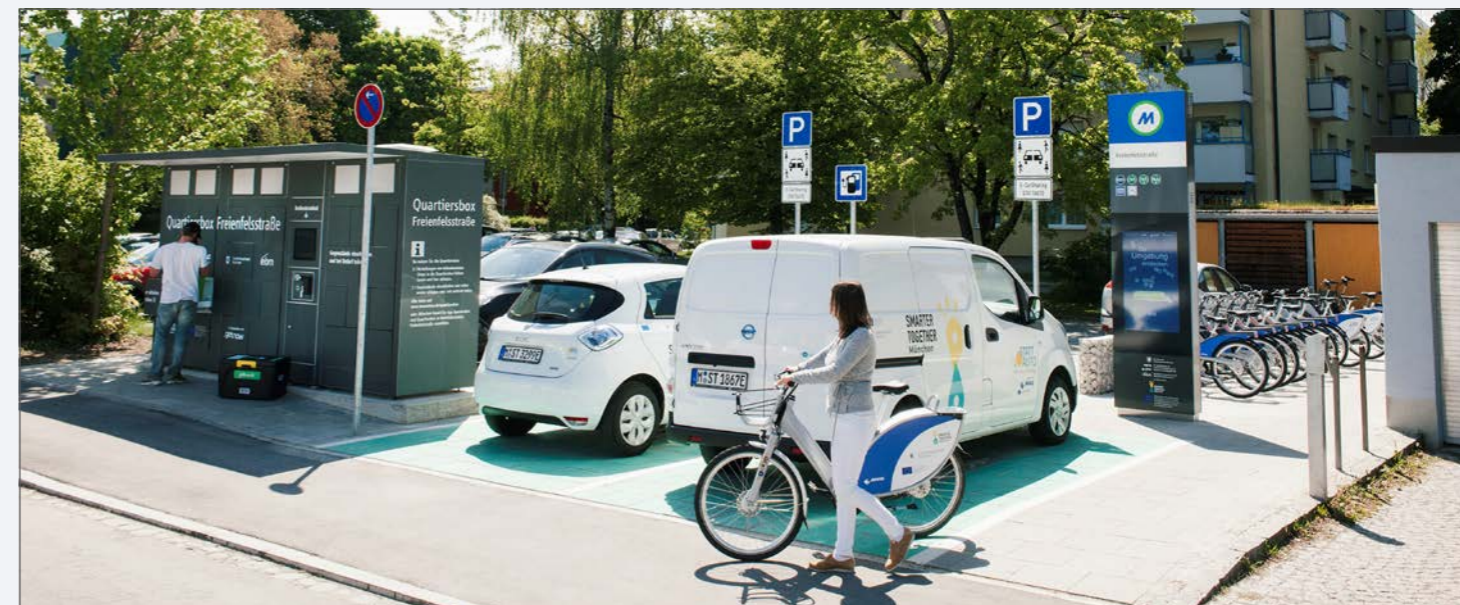
Mobility Hub Example showing electric vehicle charging, cycle hire, information board, drop off/collection facilities - Munich
