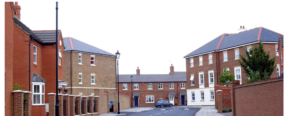
SMART Connected Community, Fairford Leys is a Live Lab for piloting a number of data and technology-driven projects.
