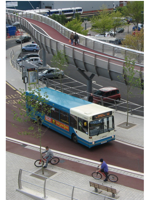
Bourg Walk Bridge
