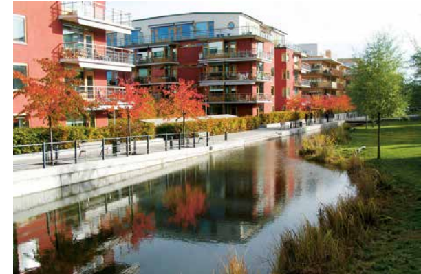
A residential-led mixed neighbourhood celebrated for sustainable design and interaction with water, Hammarby Sjöstad, Stockholm
