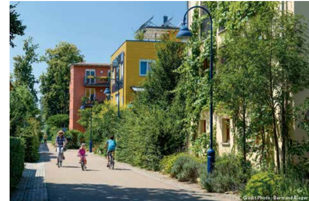
Residential-led mixed use neighbourhood which places nature and people at its core, Quartier Vauban, Freiburg
