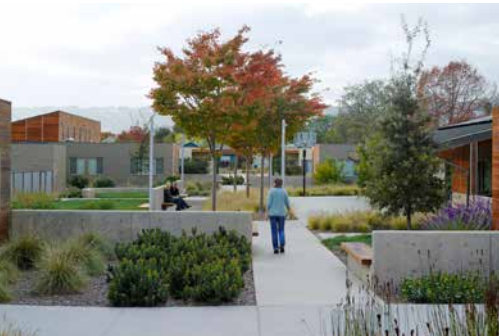
Streetwater Spectrum community, Sonoma, USA creates a public realm anchored by community facilities and designed around autism-specific principles to promote a sense of calm.
