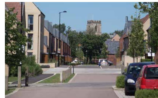
Well proportioned street framing the view, Trumpington Meadows, Cambridge
