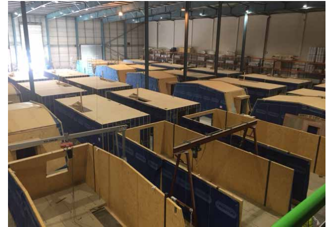
Modular construction factory, Ashford (source: Brooke Homes)
