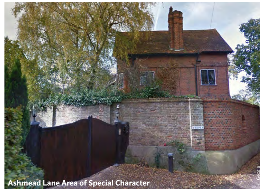
Ashmead Lane Area of Special Character
