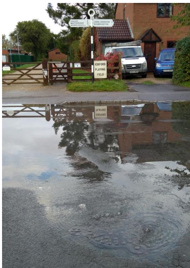
Figure 8-8: Flood water and sewage emerging from manhole on Sheldon Road outside the school (taken October 2020)
