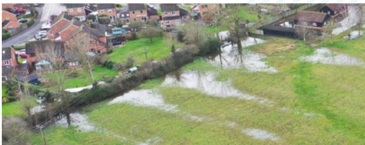
Figure 9-1: Waterlogging on the 42 Worminghall Road development site (taken December 2020).
