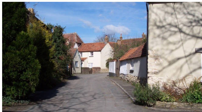
Witchert building in Haddenham
