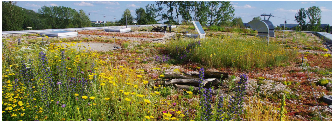
A bio-diverse (brown) extensive roof
