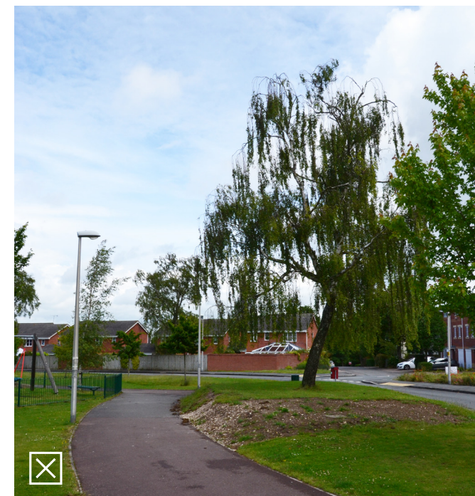
Levels and grading around an existing retained tree were poorly resolved leaving the tree on an 'island'
