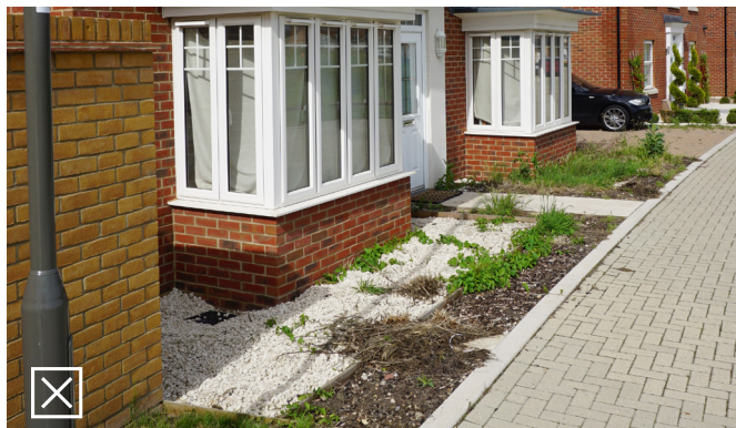
The interface of residential plots with the footways should be defined by a boundary that responds to the context
