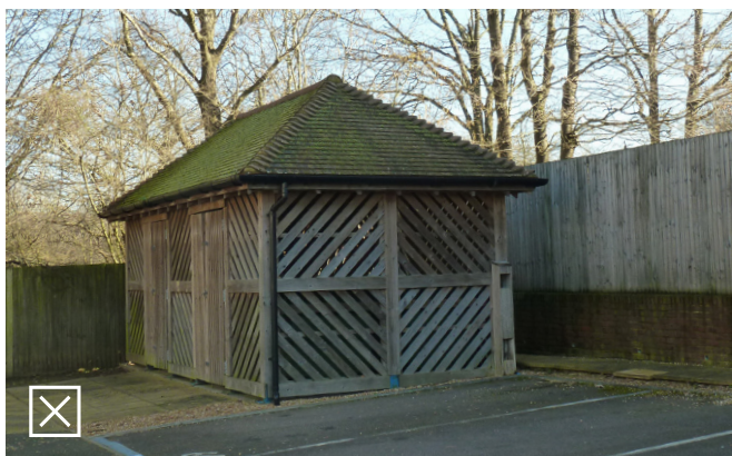
Bin stores is located within parking spaces and appears to be an afterthought
