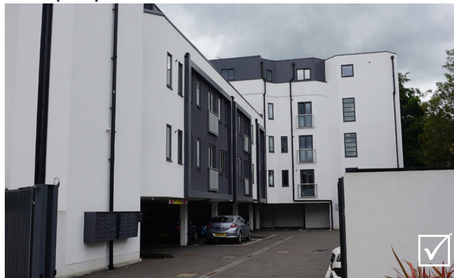
Conversion of Ringwood House, Aylesbury, from office to residential use - car parking is within an undercroft where it is hidden from the street
