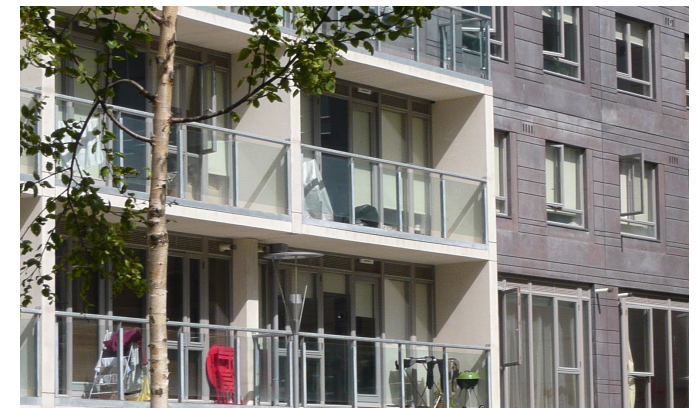
Recessed balconies provide additional privacy to the rooms that open onto them
