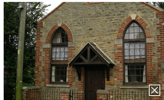
Internal floor division is visible through window
