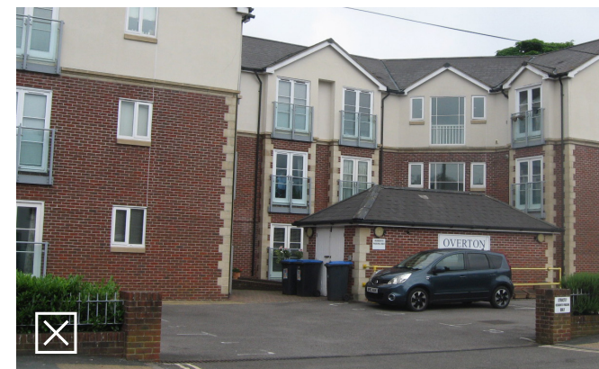
Bin store obscures building frontage and presents a poor outlook from properties
