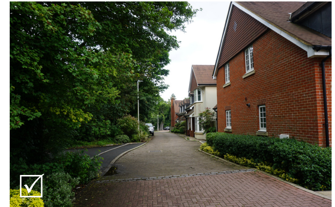
Homes at the former Princess Mary's hospital in Wendover have a positive relationship with the adjacent woodland
