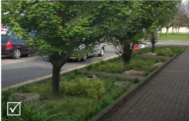
Storm water rain gardens can be incorporated within the street design to attenuate rainwater
