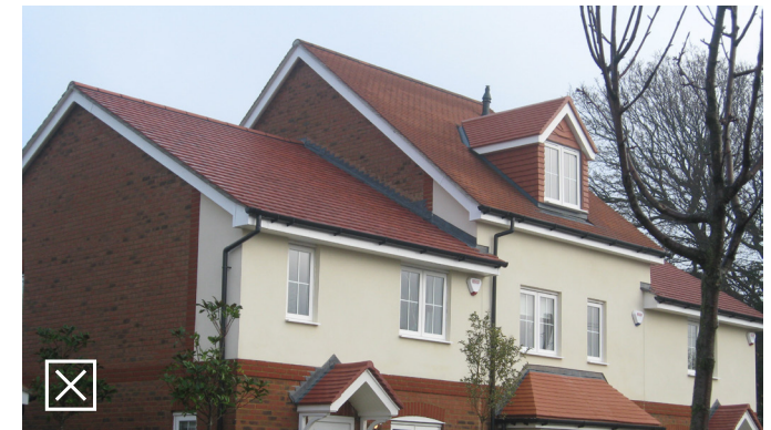
Clumsy juxtaposition of properties with inconsistent roof angles / over-dominant roof dormers
