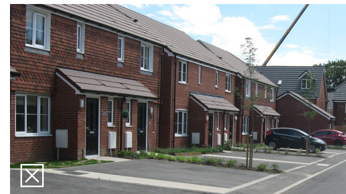
Meter boxes are prominent on building frontages
