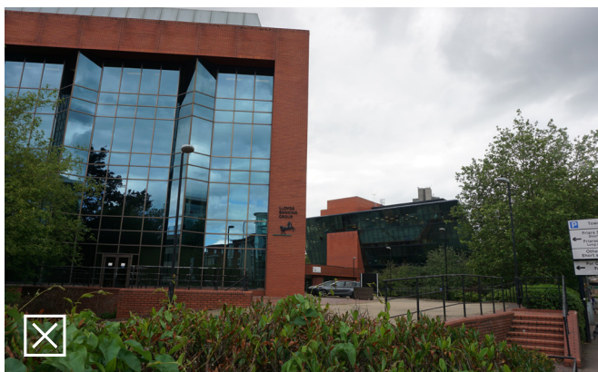
Office building is set back from the street and the entrance is not obvious
