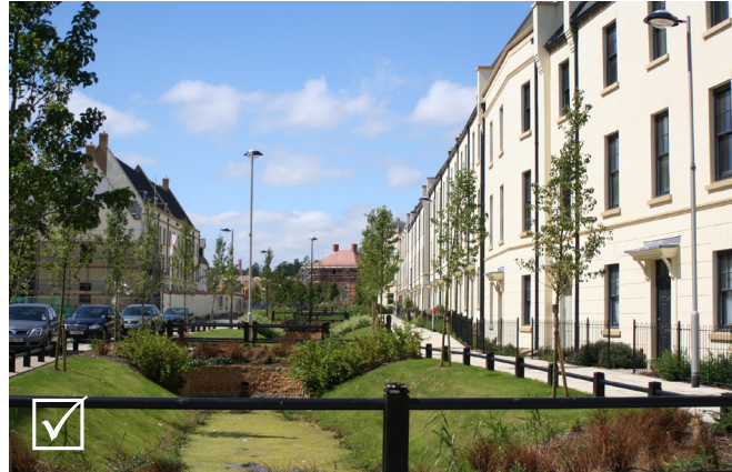
SuDS feature integrated within the streetscene in Upton, Northampton
