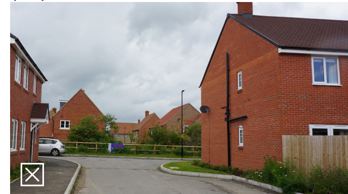
Waste pipes are prominent on the gable facing the street
