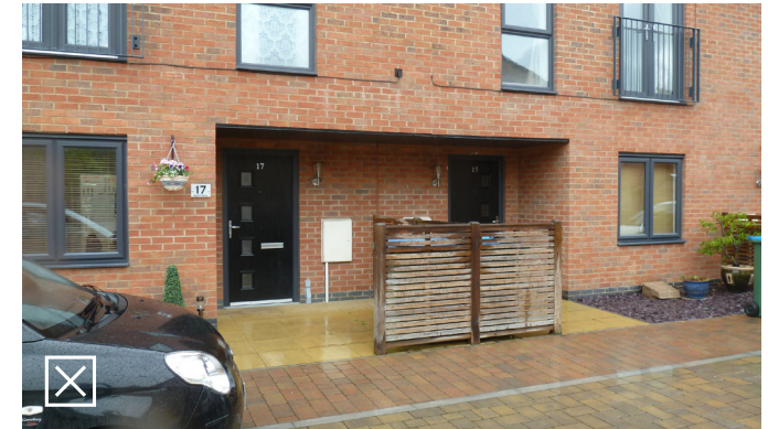
Defensible space provided at entrance to properties but materials lack robustness
