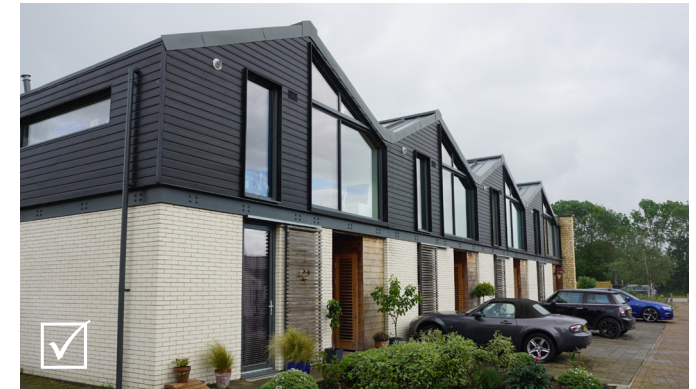
Roofscape at Marsworth Yard contributes to an industrial waterside aesthetic
