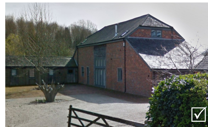
Successful retention of existing openings
