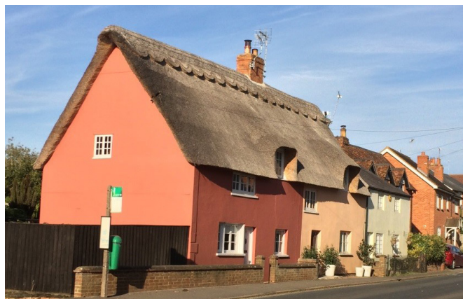
Varied roof pitches and materials, including thatch, tiles and harmonious coloured lime washed render
