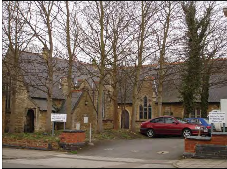
Figure 29: Former School, St James' Street
