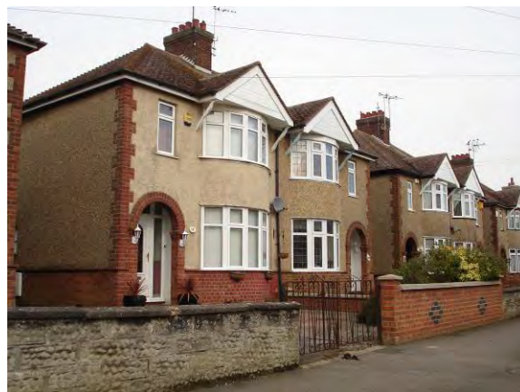
Figure 24: Late 1920s/1930s Housing, Gloucester Road
