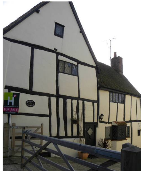
Figure 28: Close-studding at 53 High Street
