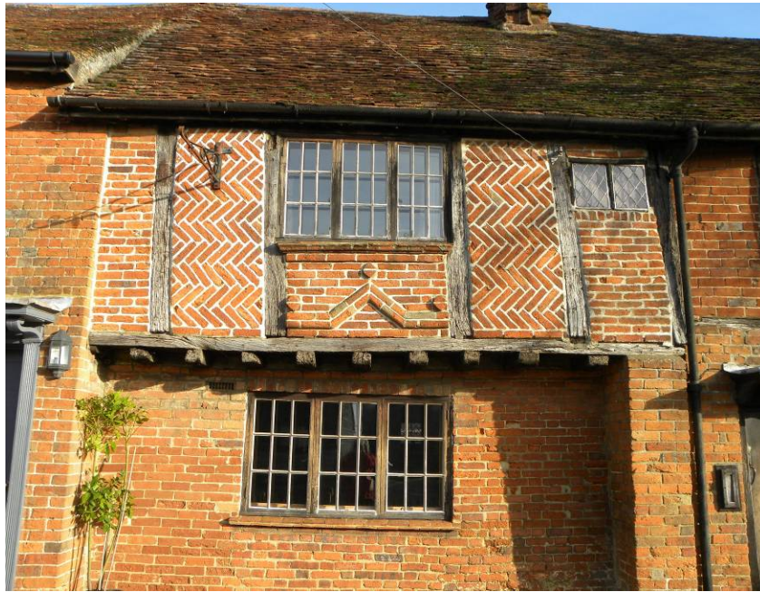
Figure 29: Brick nogging and jetty at 28 High Street
