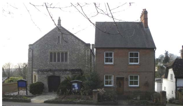
Figure 33: Methodist church and former manse
