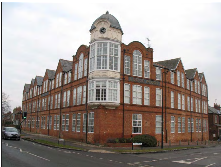
Figure 21: Hines/Lodge Plugs Factory, Wellingborough Road
