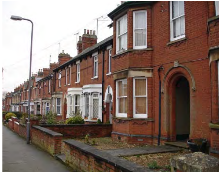
Figure 22: Edwardian terraced housing, Midland Road, Olney
