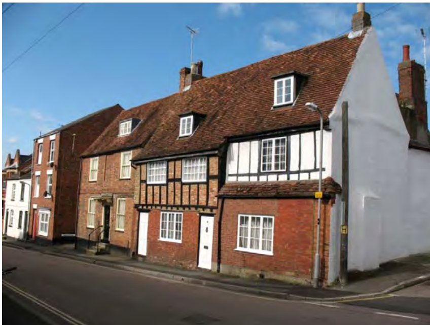
Figure 22: Timber framed jettied buildings, 16 to 18 Silver Street showing later under-building beneath the jetties extending the building forwards,
