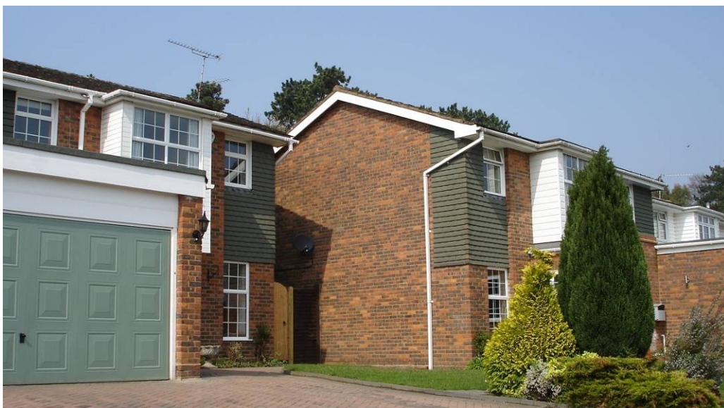
Figure 37: Housing at Terrington Hill, Marlow
