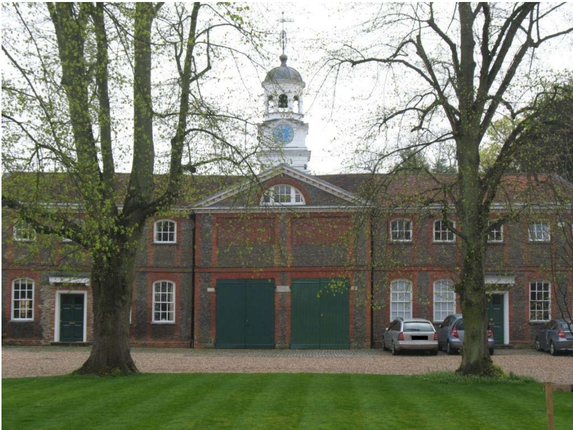
Figure 38: Remnantz, Former Military College, West Street
