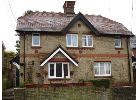
Figure 28: Some 19th century houses
