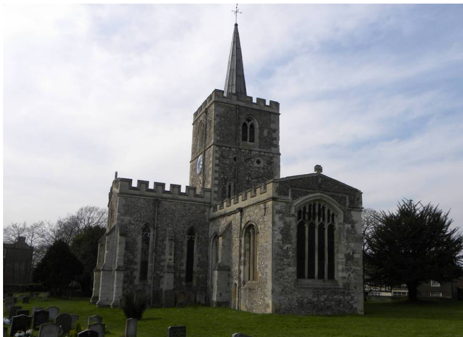
Figure 14: St. Mary's parish church
