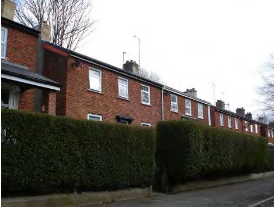
Figure 50: Steel framed council houses, Orchard Road
