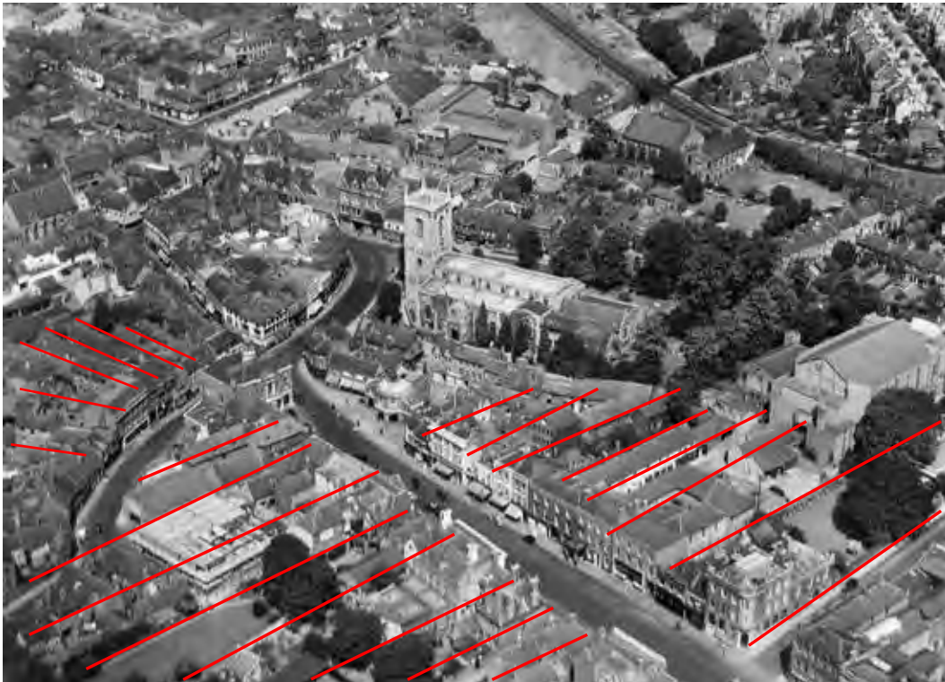
Figure 27: Aerial photograph of High Wycombe in 1937, overlaid with a graphic indicating the layout of medieval burgage plots. © English heritage – Britain from the Air
