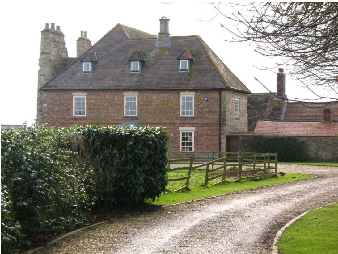
Figure 18: Old Manor House Farm (formerly Rectory Farmhouse)
