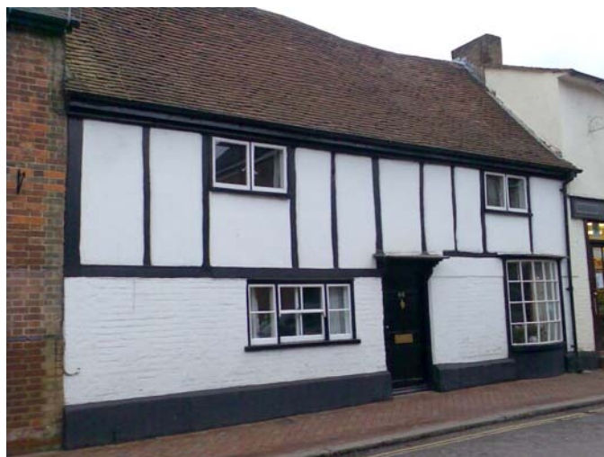
Figure 19: late 16 th /17 th century box framed building, at No. 46 High Street Great Missenden
