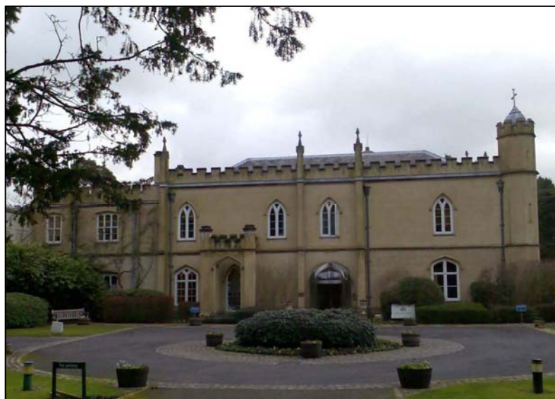
Figure 27: Missenden Abbey immediately after the fire, only the façade survived
