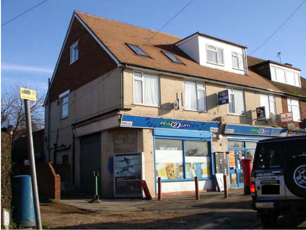
Figure 26: Shops at 1-3 Oxford Gardens
