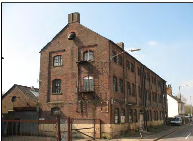
Figure 22: Hayes Boot and Shoe factory at Waterside
