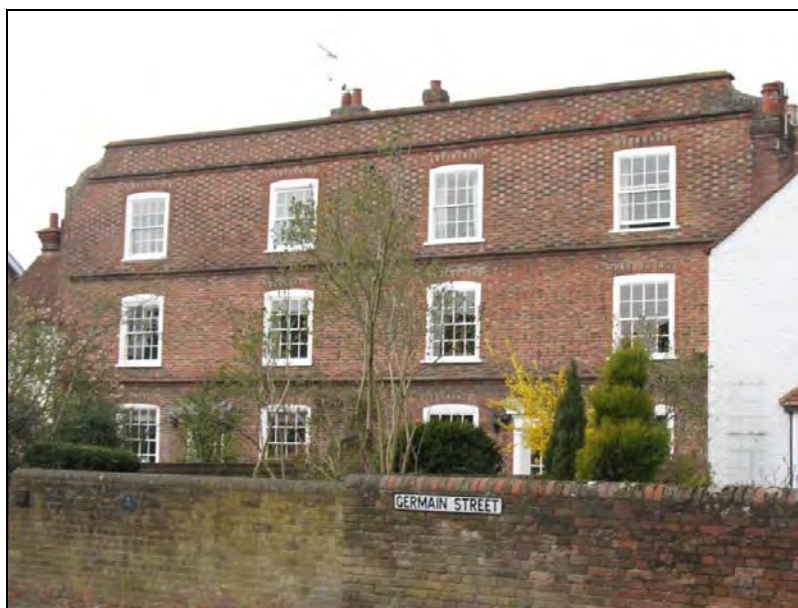
Figure 20: Weylands, German Street, former workhouse
