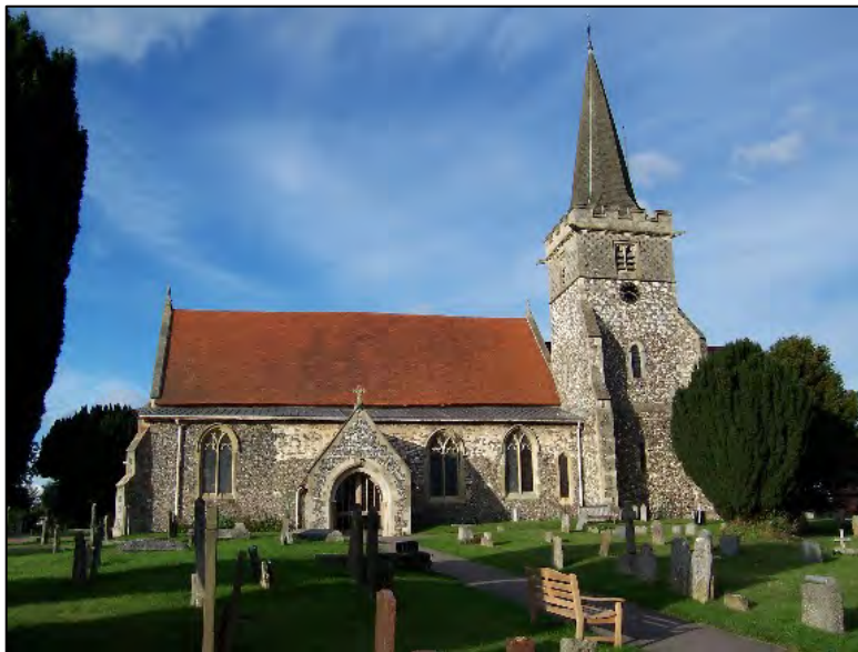
Figure 13: St Peter's Church
