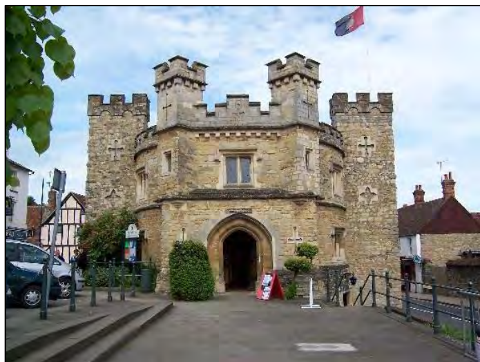
Figure 28: Old Gaol, High Street
