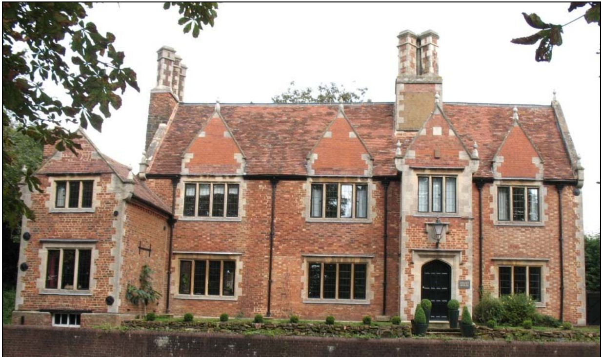
Warren Farmhouse, Little Brickhill
