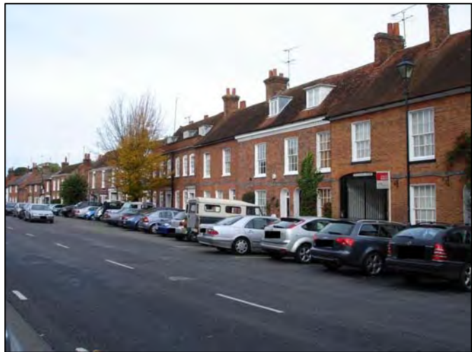
Figure 18: High Street (North) 99-133
