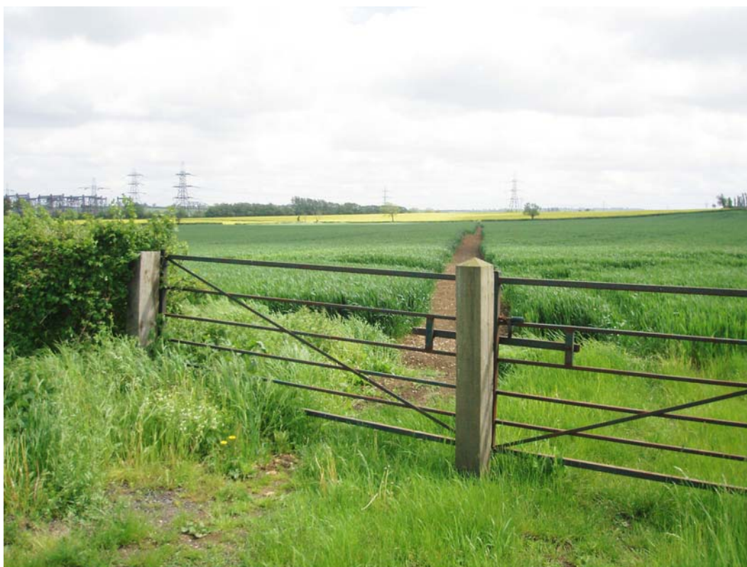
The western end of the valley includes pylons converging on the electricity sub-station visible to the left.
