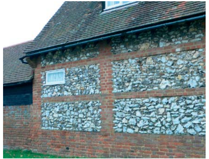
Brick and flint is a vernacular building type.
