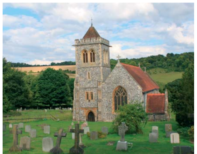
Traditional materials include brick, flint and red slate, such as at St Michael and All Angels Church at Hughenden Manor.
