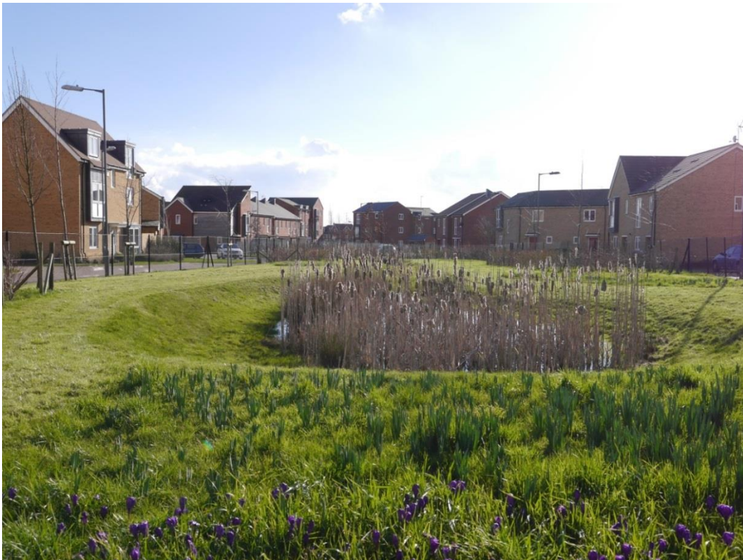
Use of an attenuation basin in Sustainable Drainage System (SUDS)
