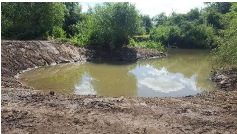
Photo 7 A newly established backwater connected to the main river channel providing new habitat for invertebrates and fish. Photo credit: River Thame Conservation Trust.
