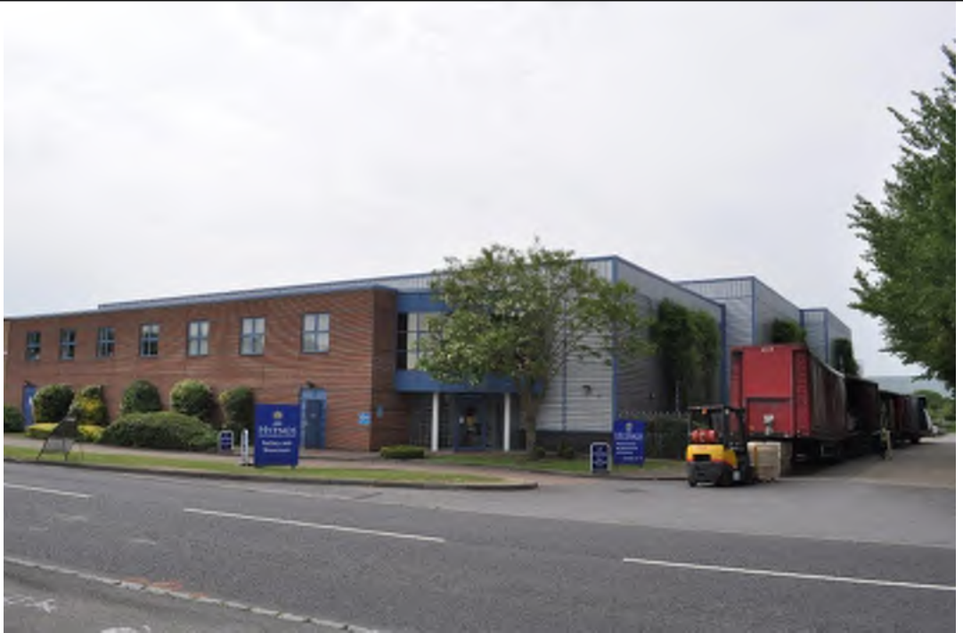
Photograph 1: Hypnos Factory and Showroom, along the bottom of the A4129 near Princes Risborough and looking west into the parcel.
