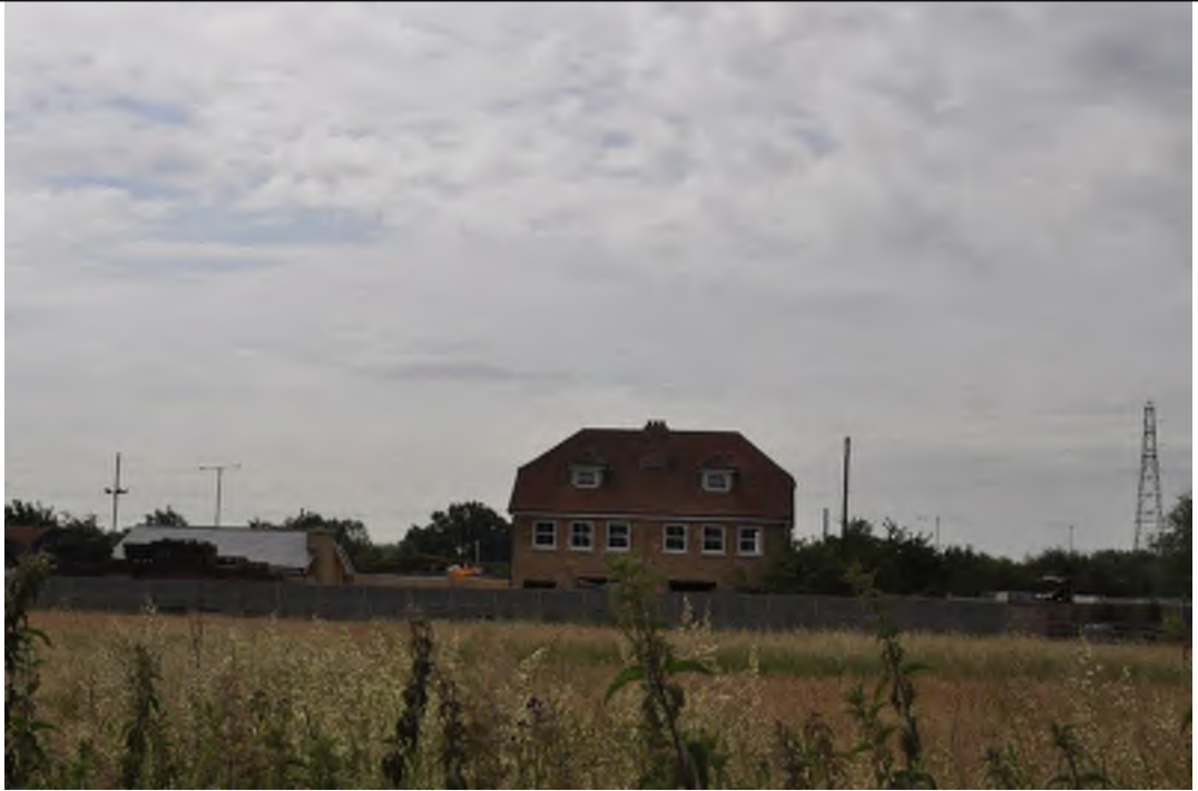
Photograph 1: View into General Area 92 from Marina Way; looking south.
