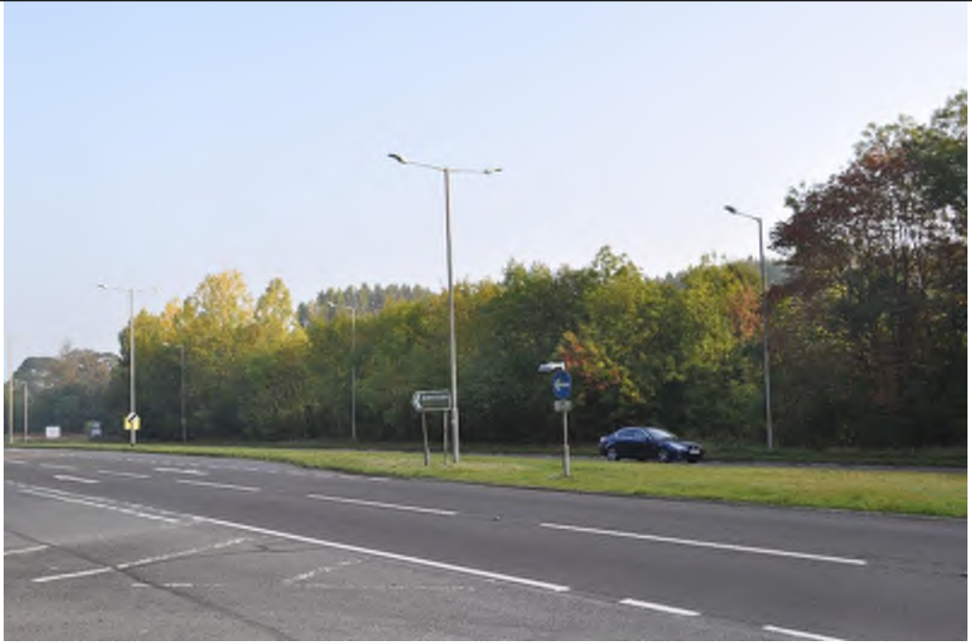
Photograph 1: View of the western edge of the land parcel, looking north-east from the junction of the A413 (Amersham Road) and South Park.
