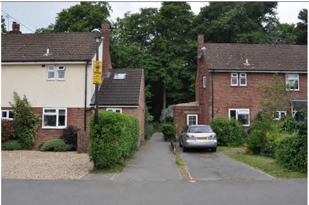
Photograph 2: View of built form and woodland behind which is characteristic of the north-west of the land parcel around Walters Ash.
