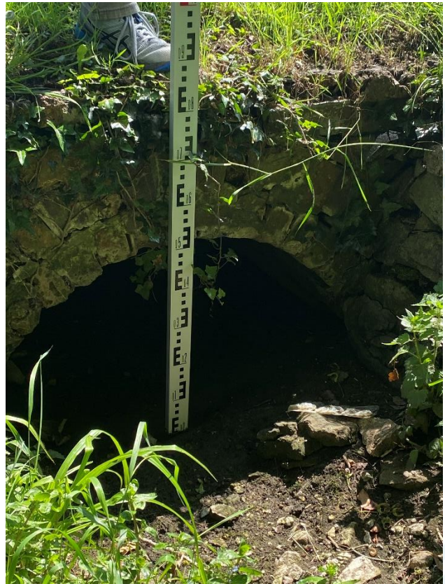
a. Figure 10-1: Channel condition around the Bridge Cottages culvert inlet (a); and Bridge Cottages culvert outlet (b).
