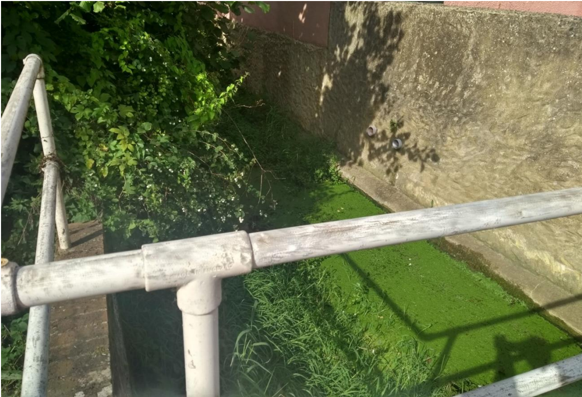
Figure 9-4: Tonne Brook on Bridge Street, September 2021
