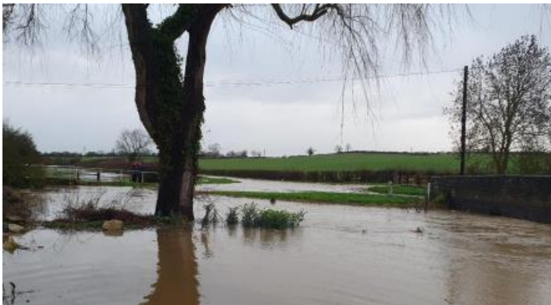
Figure 8-2: Photo of flooding at Lower End Bridge and Hatchet Leys Bridge (Locations 6 and 7), taken at approximately 16:00 on 23 December 2020 from the left bank of the watercourse. Credit: Thornborough residents
