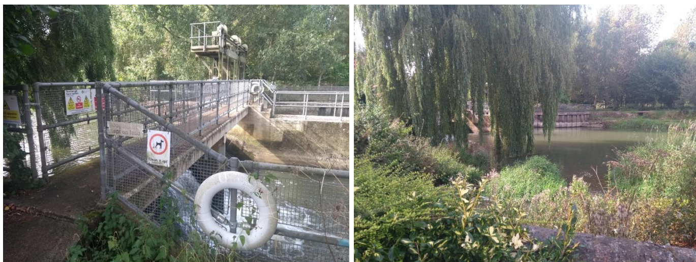
Figure 9-7: Weir on the Great Ouse at Thornborough Mill, September 2021
