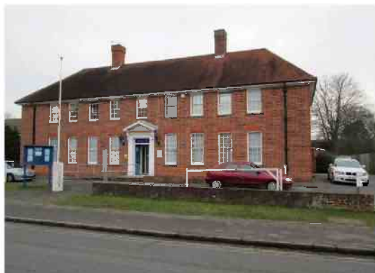
Police Station on Dean Street (with low threshold)
