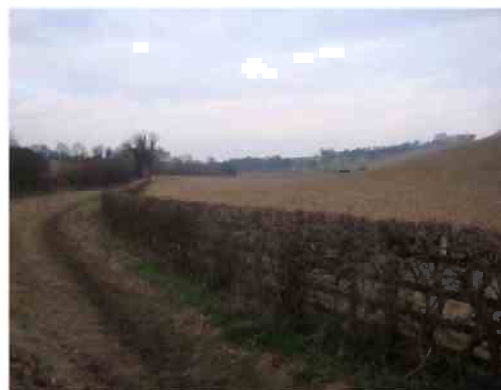
Dry valley with potential for upstream storage
