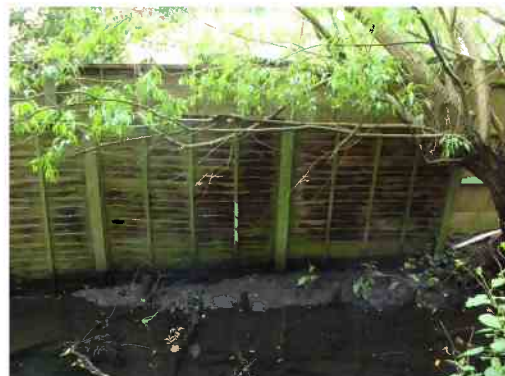
Properties on The Croft have been affected by high levels in the Newt Ditch
