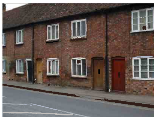
Chapel Street cottages have very low thresholds
