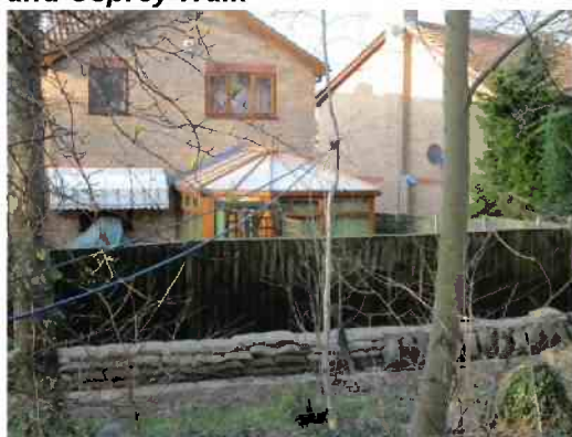
Property level protection effort to the rear of a house on Osprey Walk
