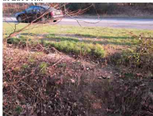
Roadside ditch by A421, with some evidence of water outflow towards houses on Osprey Walk in the foreground
