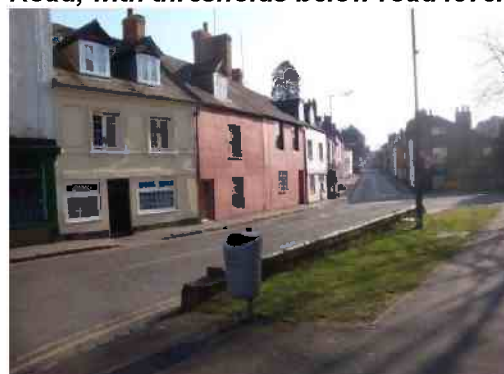
Depression near the junction of Nelson and Hunter Streets, with low thresholds
