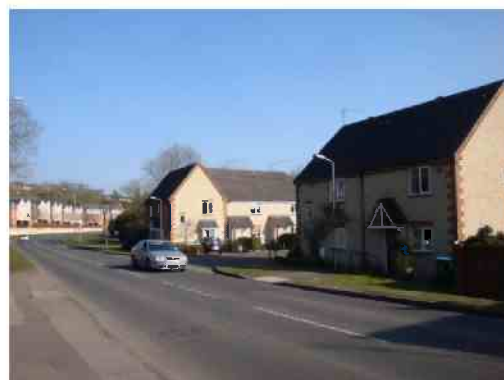
Houses in a depression on Stratford Road, with thresholds below road level
