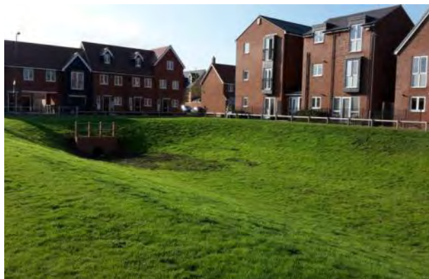
Implementation of a water storage basin as part of a sustainable drainage system, in Berryfields, Aylesbury.
