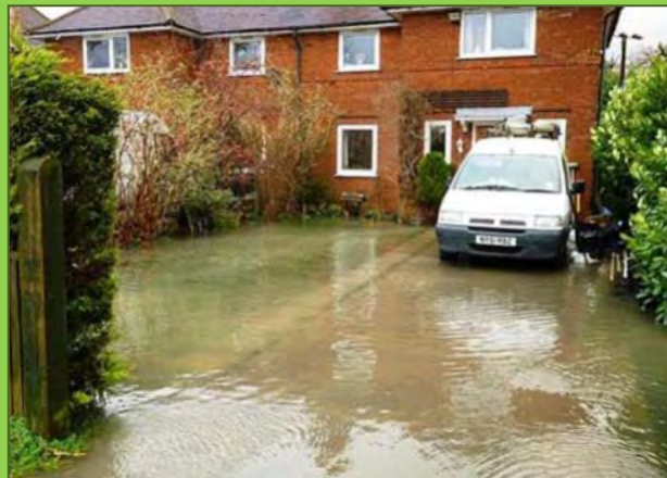
Image taken from Mill Lane, Monks Risborough S19 Flood Investigation Report
