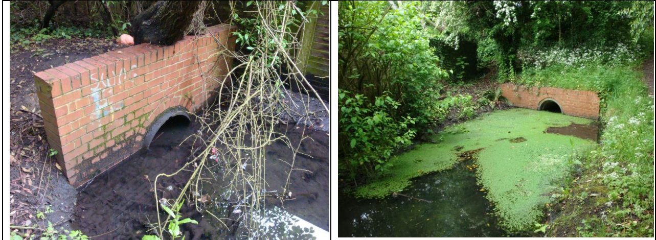
Figure 10 Newt Ditch culvert (29-05-2013)
