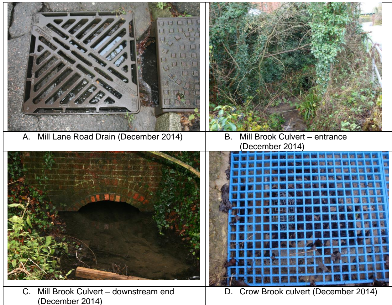
Figure 8 Condition of structures
