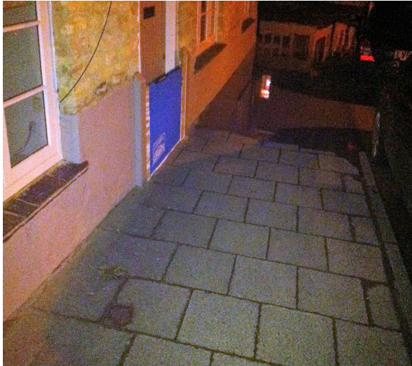
Ford Street, Buckingham at 12.15am, 10 th March 2016. Property level flood protection board (blue barrier) in operation (photo provided by Buckingham Flood Action Group).
