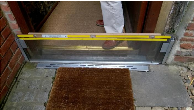
Deployed barrier at Amersham museum
