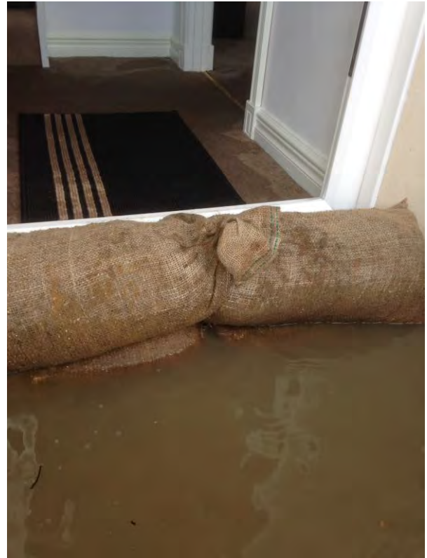
07/02/2014 12:24 Internally flooded property - Councillor Steven Lambert
