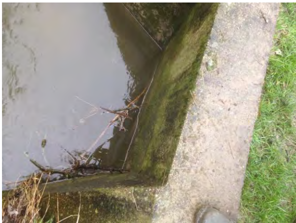
10/02/2014 16:31 Gully outfall - Councillor Steven Lambert
