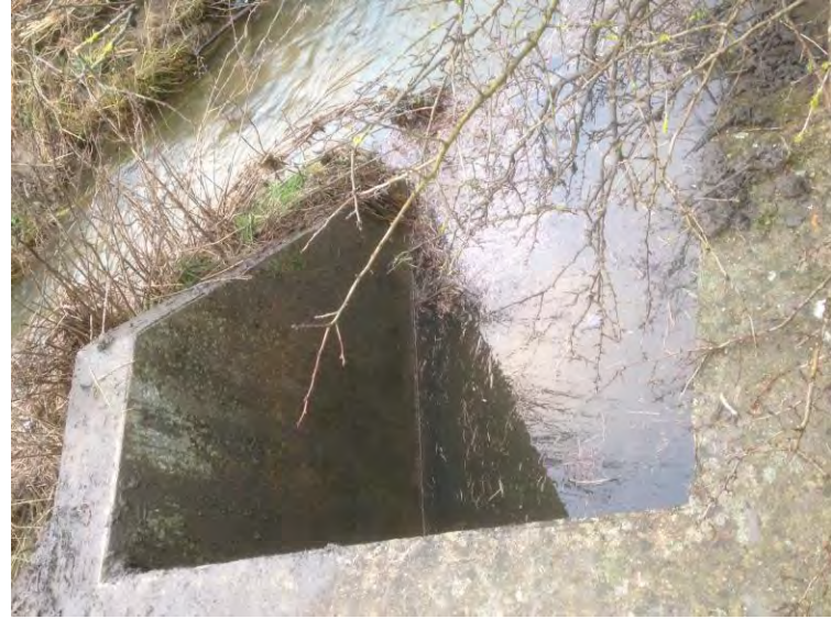
10/02/2014 16:47 Gully outfall - Councillor Steven Lambert
