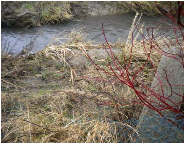
Overgrown banks with huge amounts of silt & vegetation.
