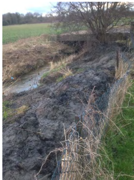
Figure 12 10/02/2014 16:52 Silt removed from Stoke Brook and gully outfall at end of Fox Glove - Councillor Steven Lambert
