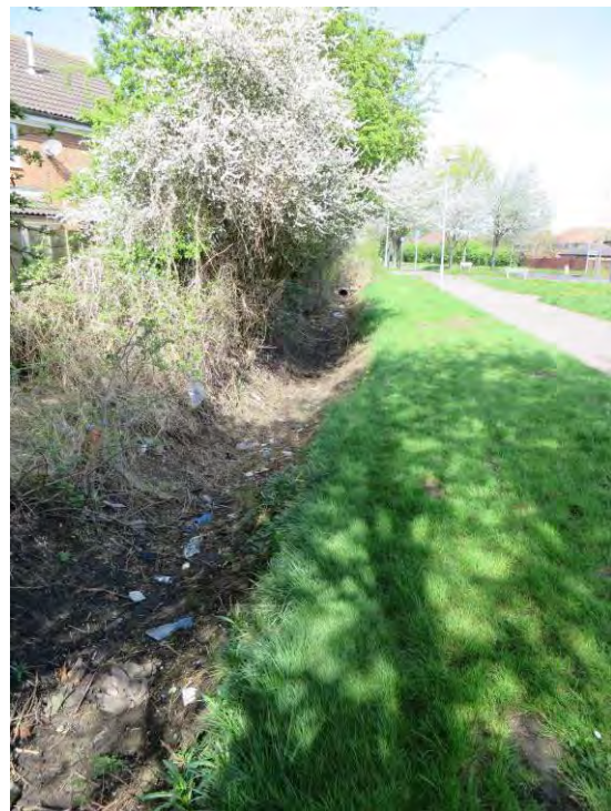
Ellen Road ditch after clearance
