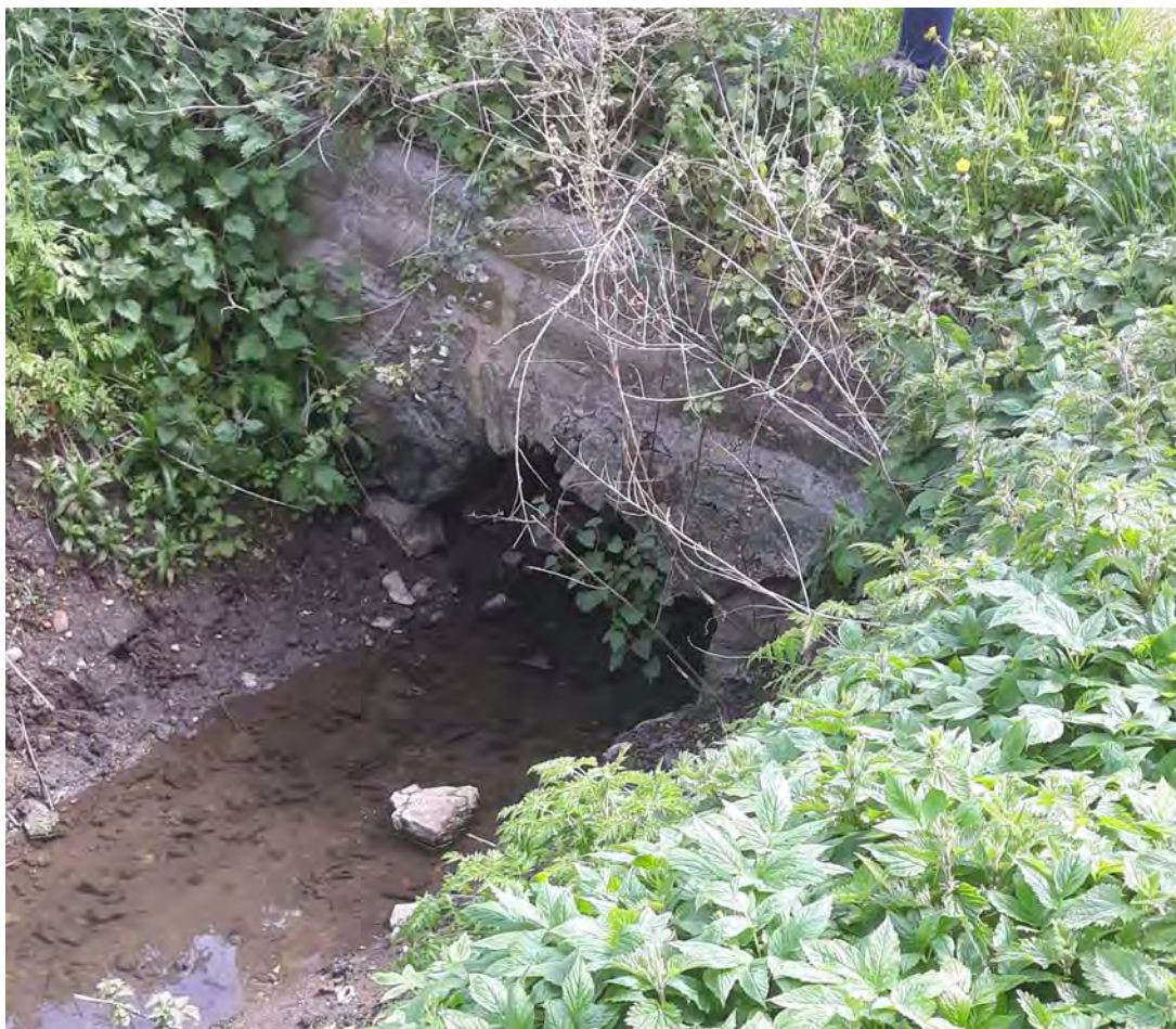
Figure 8-3: Downstream end of culvert from site visit on 6 May 2021
