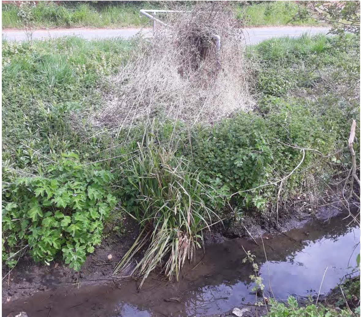
Figure 8-2: Open channel along Preston Road. Photo taken on site visit on 6 May 2021
