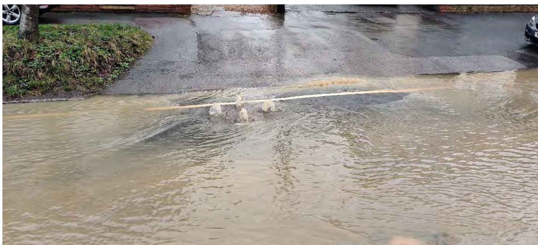
Figure 8-4: Surcharged manhole in Main Street during the event
